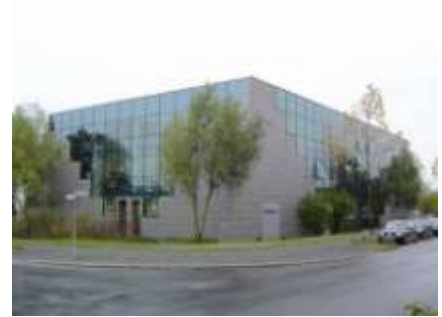
Lerros Company Building (Photo: Lerros)
